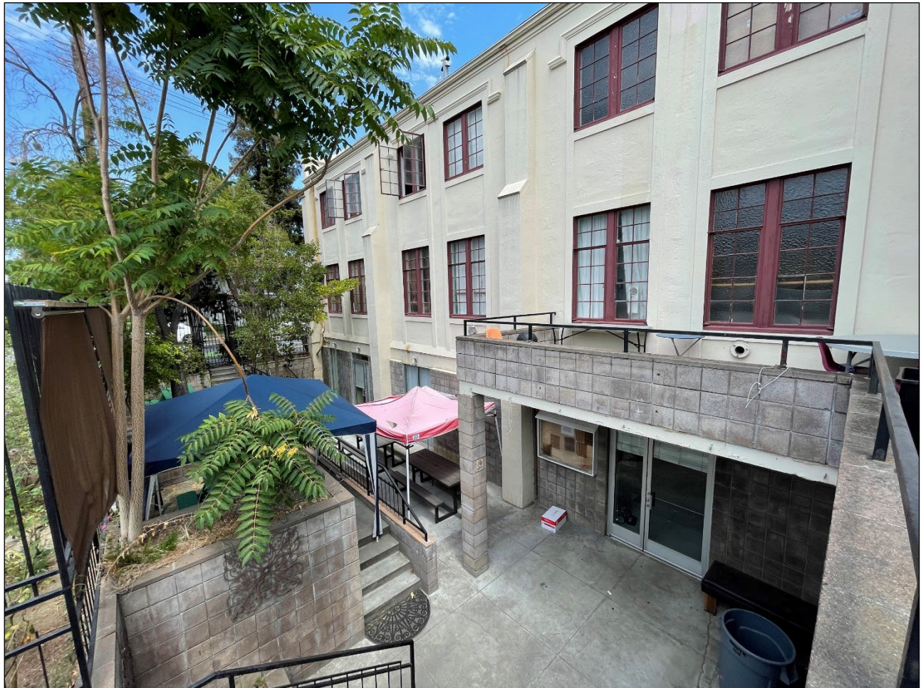
Basement level of administrative wing. This floor was modified in 1966 by excavating and creating an entrance below grade to lead into the church basement. Viewed with camera facing north-northeast.
