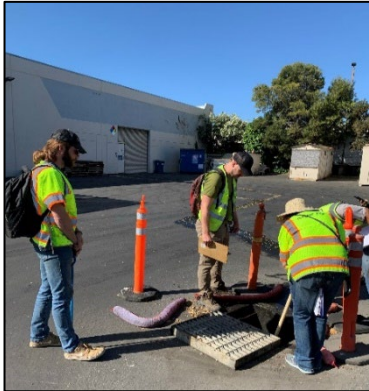
Sampling storm drain catch basins at a potential PCB source
