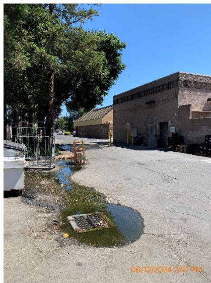
Left: IDDE case involving a water leak. Right: the leak was repaired.
