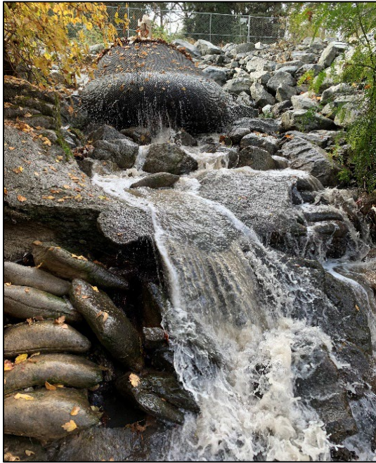
Oldcastle NetTech™ Gross Pollutant Trap (trash net) monitoring at Coyote Creek.
