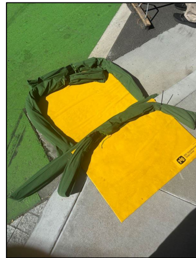
Storm drain covers and wattles being implemented by Groundwerx during pavement washing operations.
