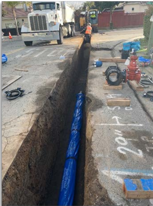
Municipal Water Main Construction Work
