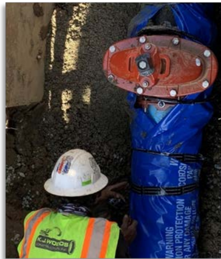
Water Valve Installation
