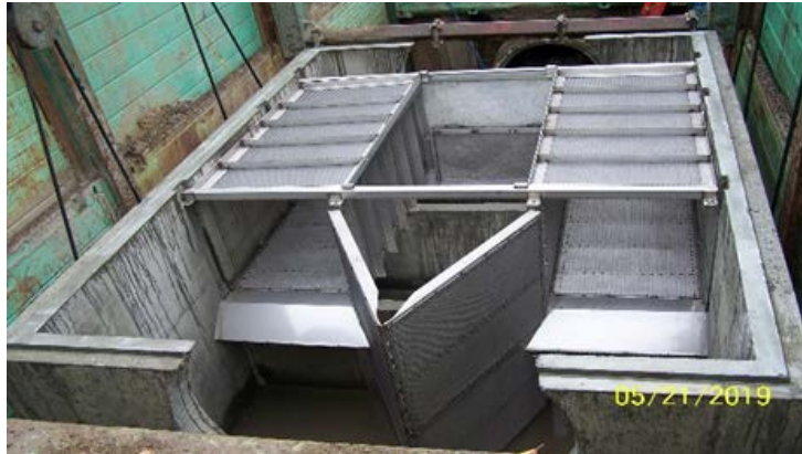
Large Trash Capture device installation
